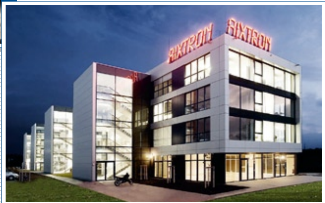
04 OFFICE COMPLEX IN OCTOBER 2010 //
